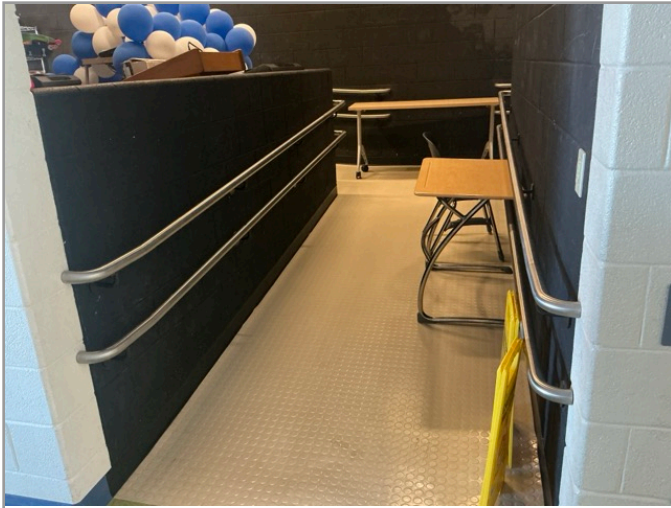
ACCESSIBLE INTERIOR RAMP
