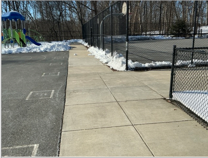
ACCESSIBLE ROUTE TO PLAYGROUND
