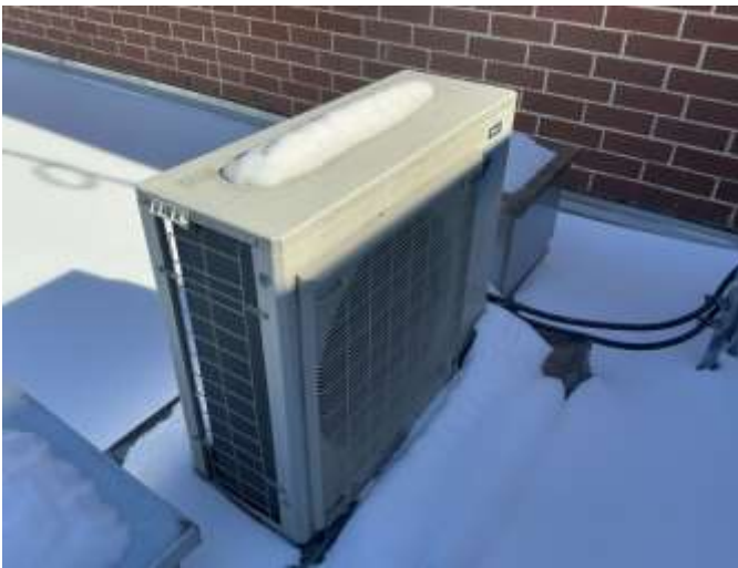
21 - SPLIT SYSTEM DUCTLESS
