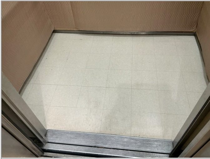
LOBBY LOOKING AT CABS (WITH DOORS OPEN)
