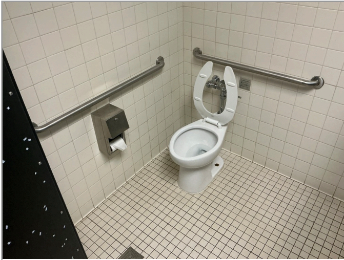
TOILET STALL OVERVIEW
